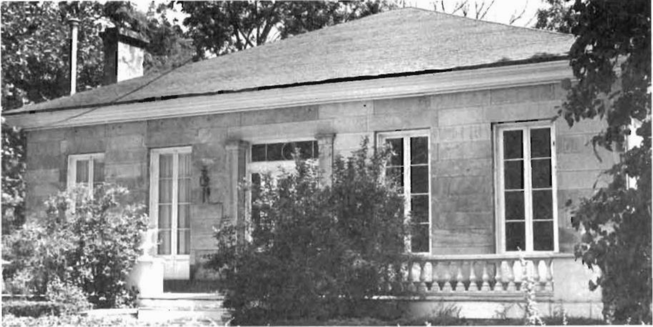
38. Woodale, 35 Cross Street, Dundas, Ontario; Constructed 1841; Material stone.
