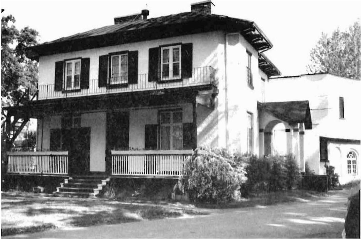
70. Sunnyside, 239 Union Street, Kingston, Ontario Constructed ca. 1841-42; Material brick and stucco.
