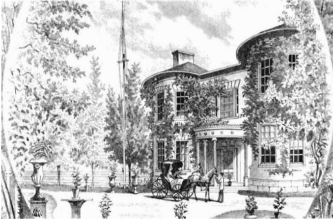
112. Fairholm in the Nineteenth Century, 230 Prince Street, Charlottetown, Prince Edward Island Constructed 1837-40; Material brick.
