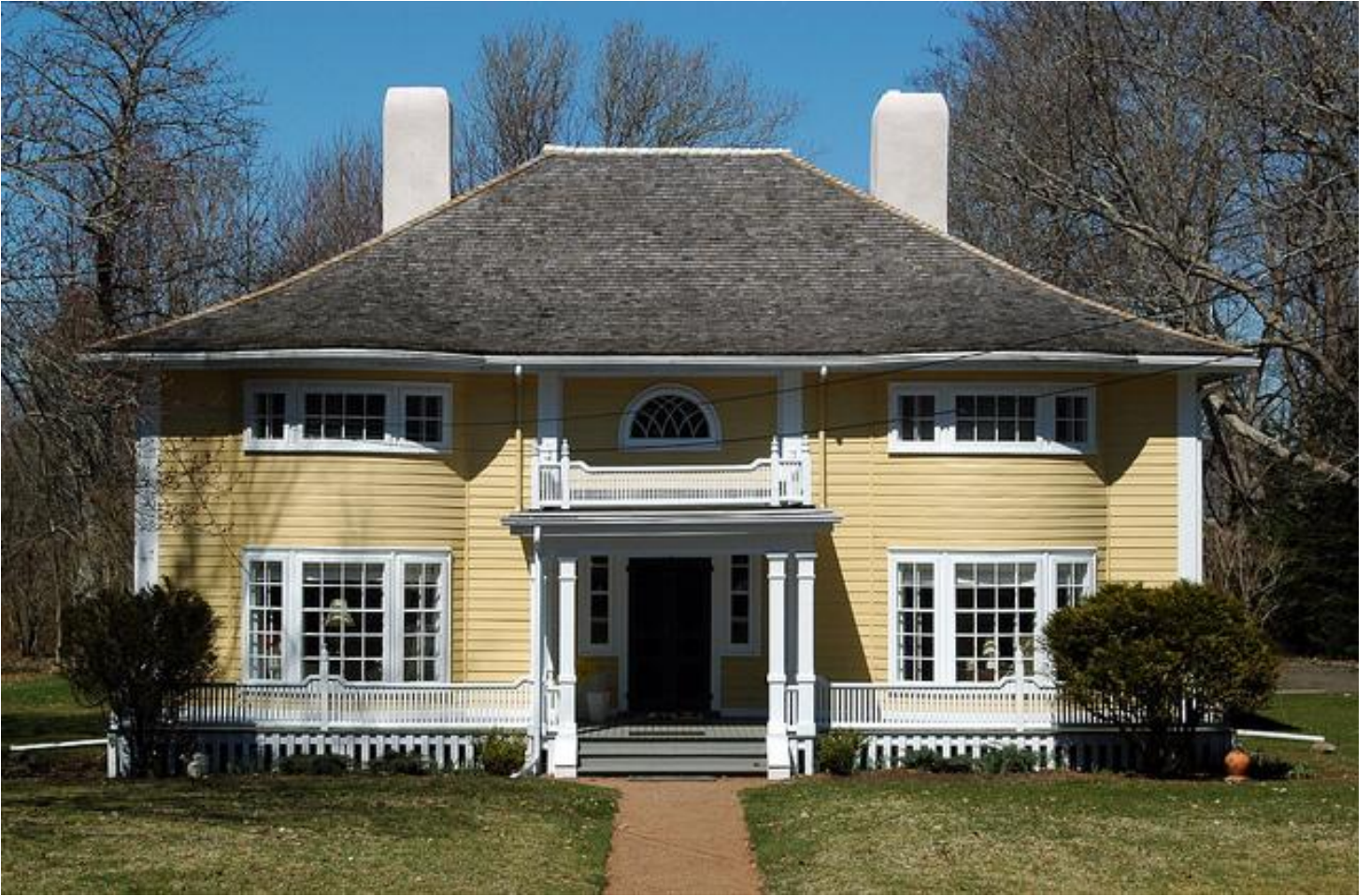
110. Girvan Bank , 478 Saint George Street, Annapolis Royal, Nova Scotia Constructed 1817; Material wood.
