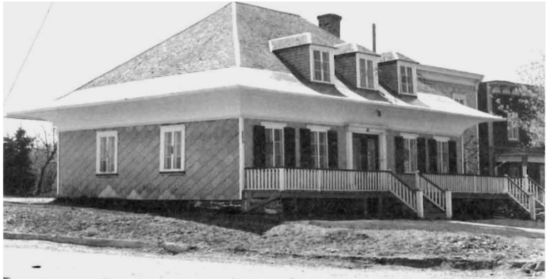
103. Cottage, 118 Saint-Georges Street West, Lévis, Québec; Material wood.
